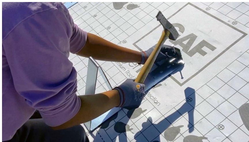
Fig. 10. – NAILING STAGER 2
