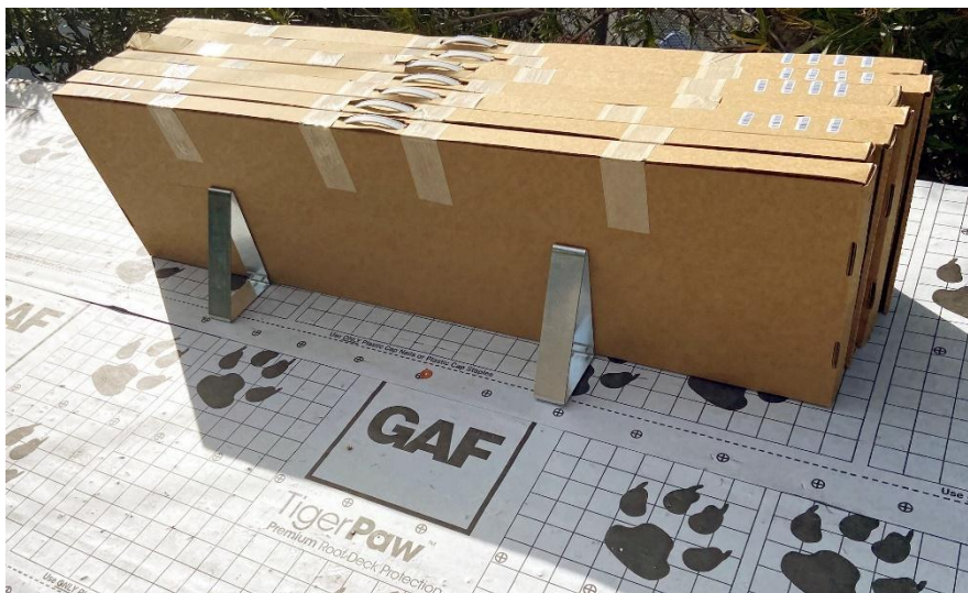
Fig. 11. – TIMBERLINE SOLAR ENERGY SHINGLES "STAGED"
