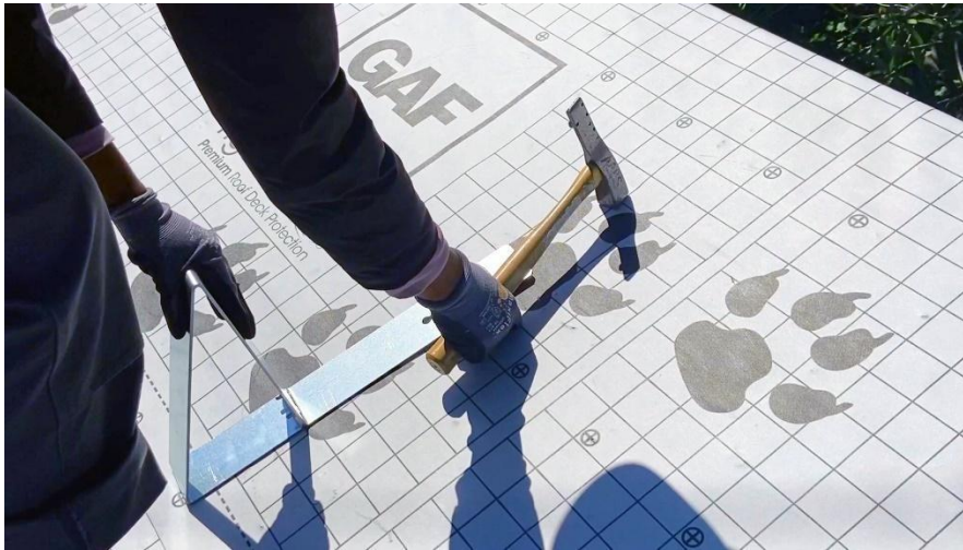
Fig. 4. – CHECKING FOR RAFTER
